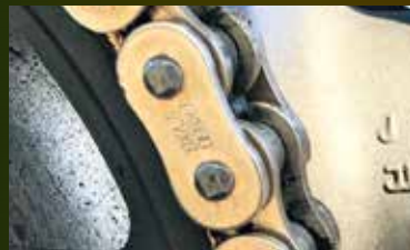
no rust, good condition
